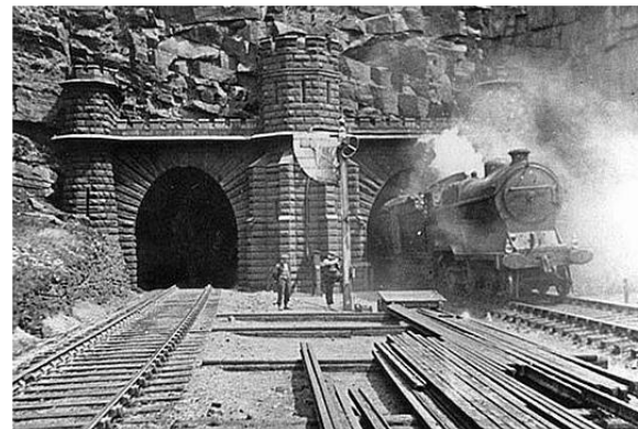
The Woodhead Tunnel - c1985
